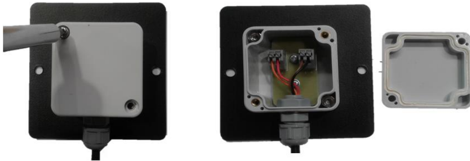
Fig. 12 – Opening the back of the wallswitch
